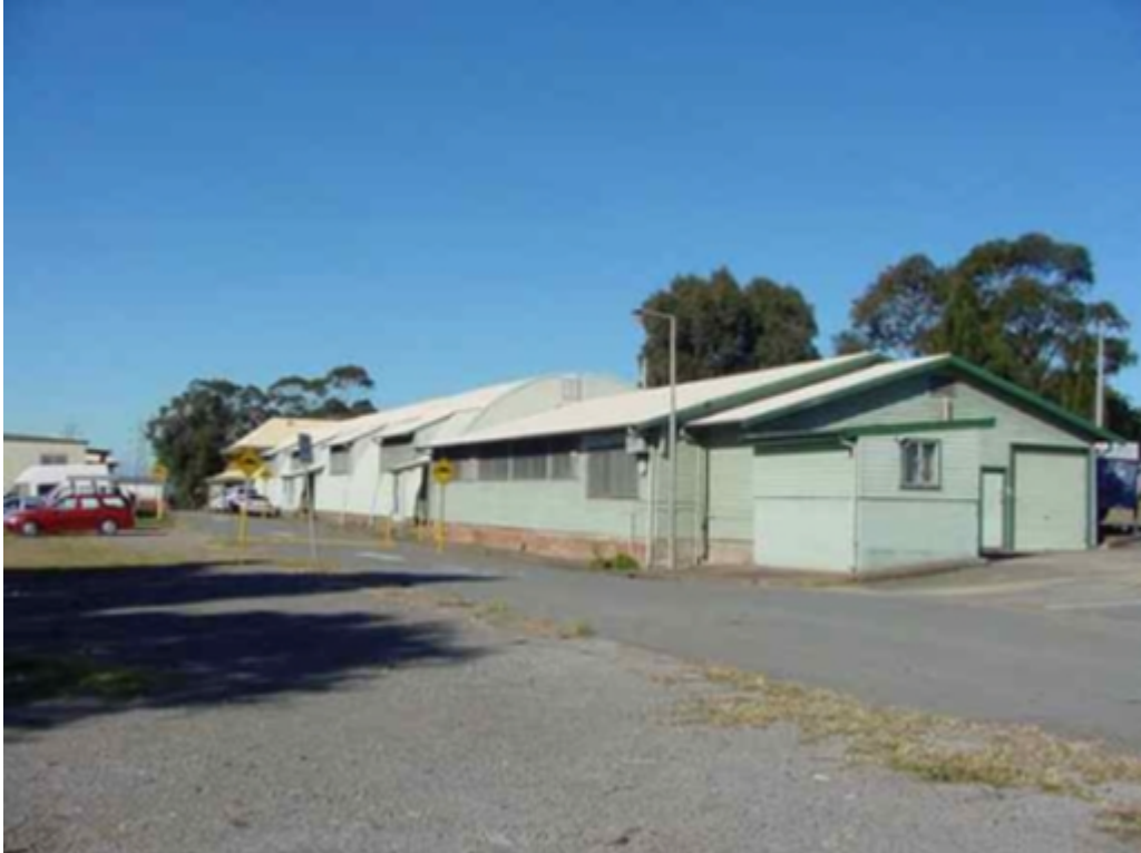
Plate 1: showing main group of buildings at the Former Migrant Camp. Small gate house in the foreground and view along the Quonset hut and pitched roofed addition. Photo taken in 2007 by Sarah Cameron (copyright NCC).
