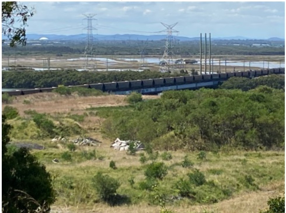
Plate 8: View looking north-west over part of the proposed Steel River Battery site on rhs. The site has since been levelled and cleared for the proposed development (Photo taken 22/10/20).
