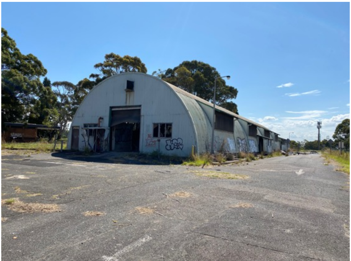
Plate 6: Current view of the east elevation – although vandalised the Quonset building remains intact
