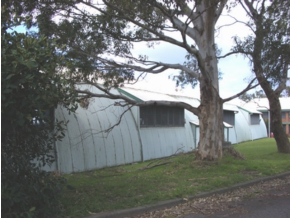
Plate 5: View along the south elevation Quonset building photo taken in 2007 by Sarah Cameron (copyright NCC).
