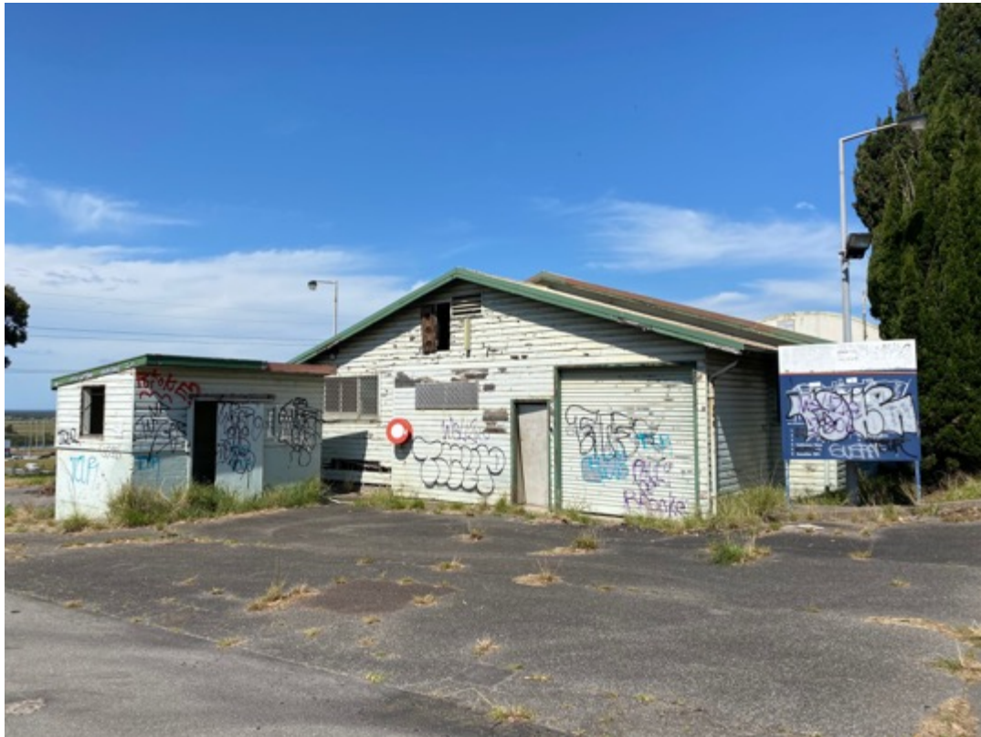
Plate 3: Current view of the west elevation including the small gate house in the foreground
